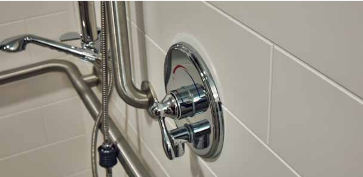
decorative shower walls
